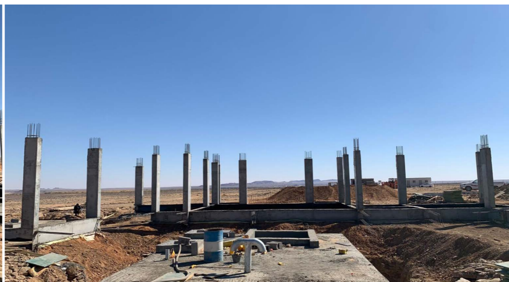
Al-Sabkha Administrative Building
